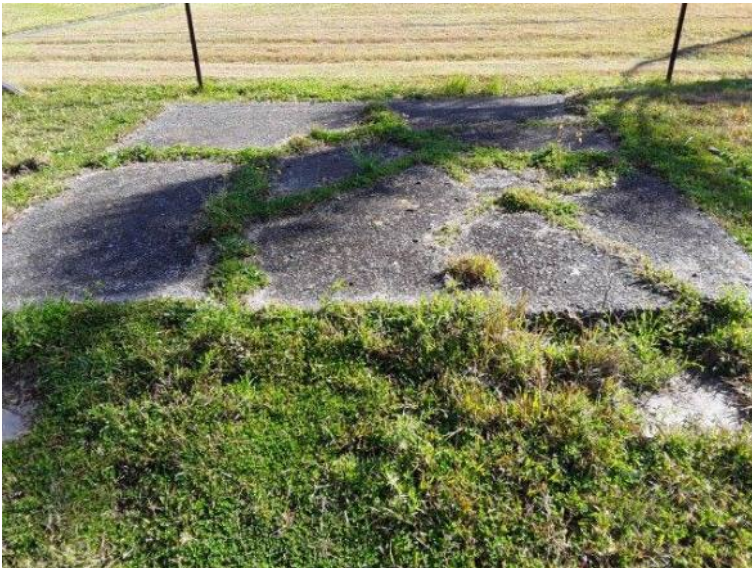
Photo 19 Concrete slab within the central portion of the study area
