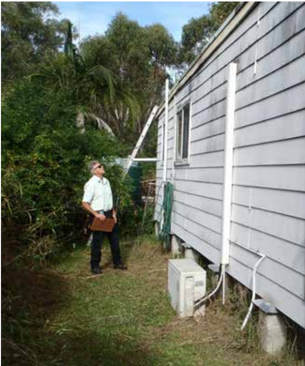
Council Building Inspectors are now assessing properties for required improvements within the subdivision.
