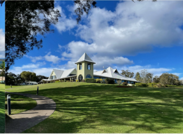
NORTH-WEST VIEW OF EXISTING FUNCTION CENTRE
