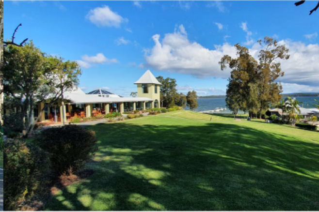
NORTH-EAST VIEW OF EXISTING FUNCTION CENTRE
