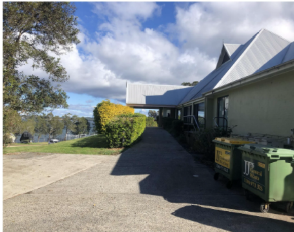
VIEW CORRIDOR TOWARDS LAKE MACQUARIE ALONG SOUTHERN EDGE OF THE EXISTING FUNCTION CENTRE
