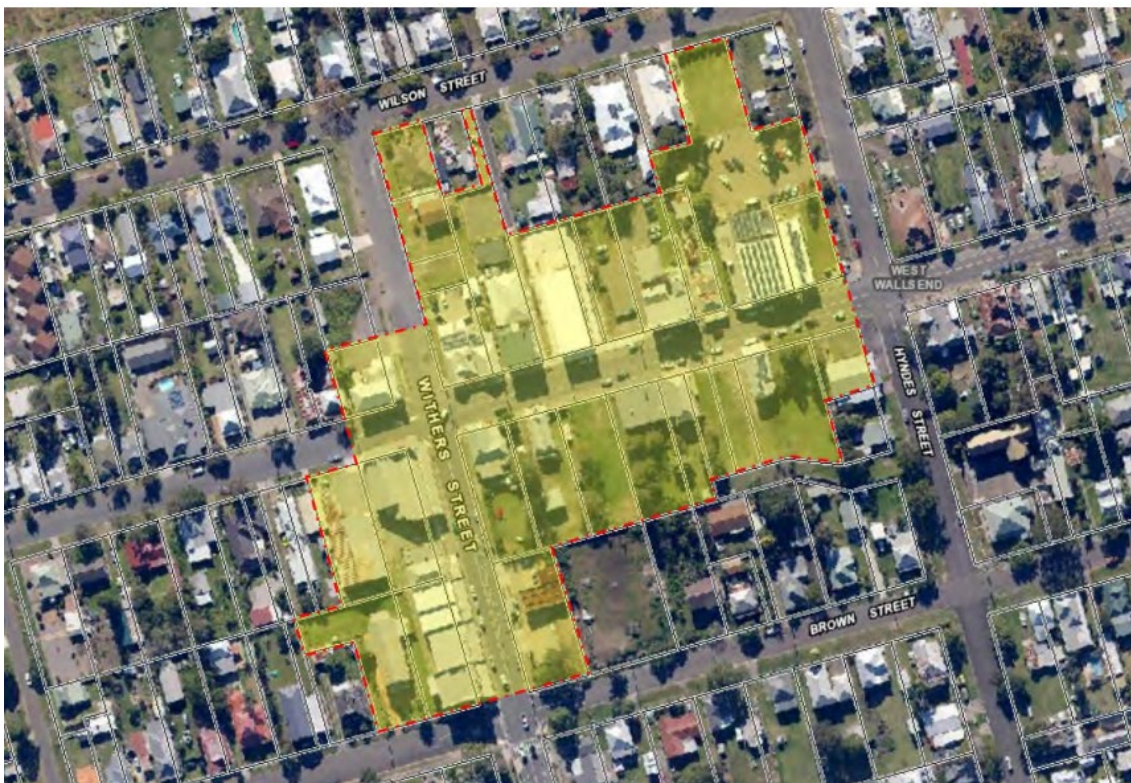
Figure 4 - The Carrington and Withers Street Axis area in West Wallsend where the height of existing development is generally greater than one-two-storey
