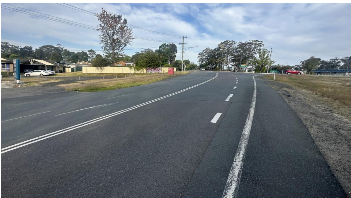
Figure 3.7: Wye Road Facing Southeast Proximate to the Site
