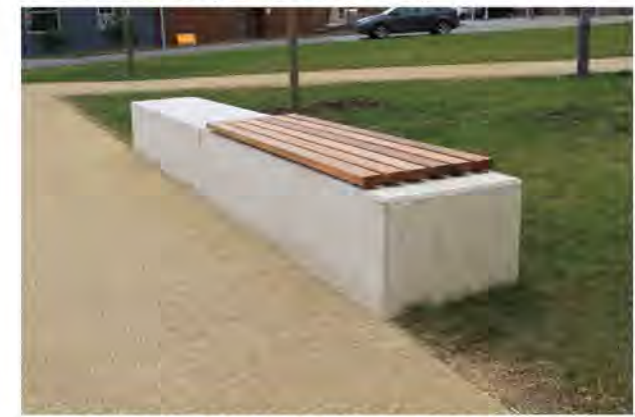
HARDWOOD TIMBER CAPPING TO BE FIXED TO TOP OF SANDSTONE LOG (STAINED TO DARK TONE)
