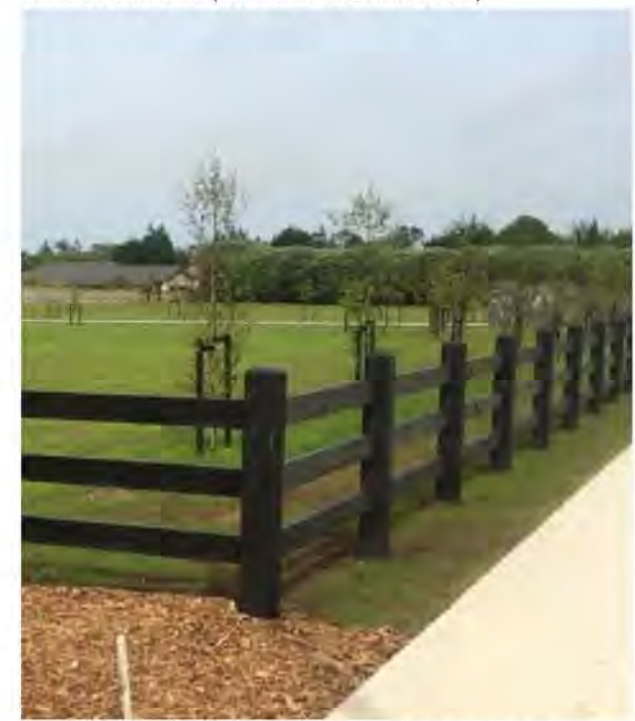
TIMBER POST & RAIL FENCE (BLACK) BOUNDING THE CEMETERY TO SURROUNDING ROADS AND PLAYGROUND.
