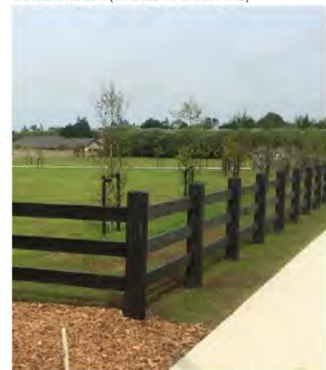
TIMBER POST & RAIL FENCE (BLACK) BOUNDING THE CEMETERY TO SURROUNDING ROADS AND PLAYGROUND.
