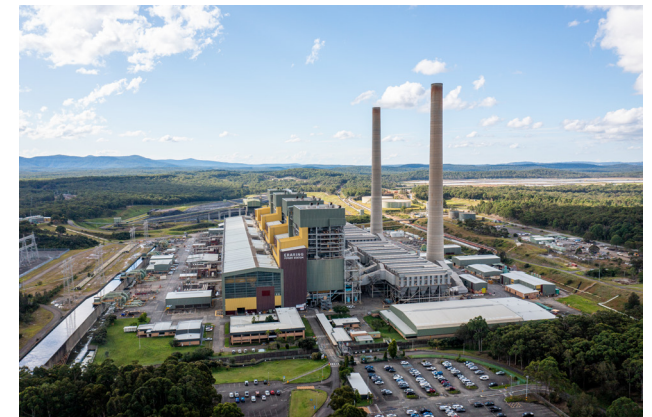
Eraring Power Station
