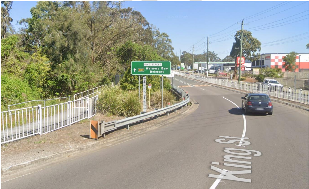
Photo 42: Flood depth indicator on King Street at North Creek ( Source: Google Street View )
