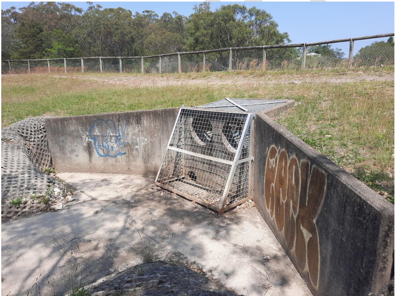
Photo 36: Debris control structure on the outlet of the Vermont Place detention basin
