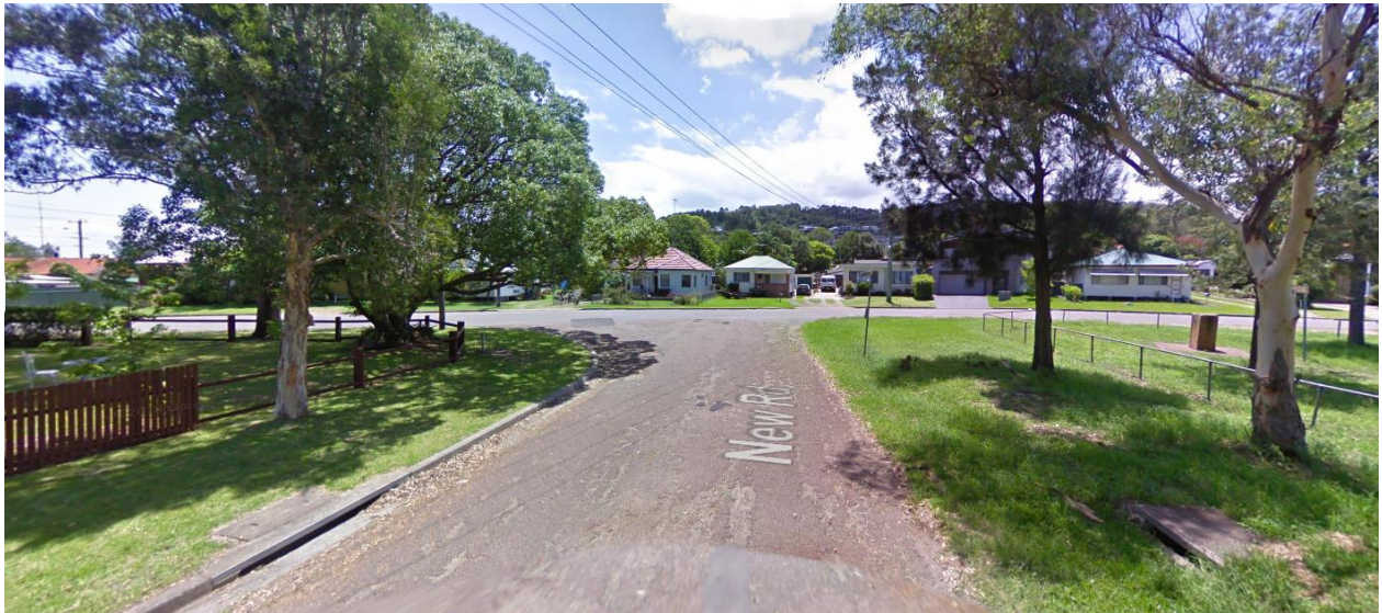
Photo 28: New Road looking west to Seaman Avenue at the low point ( Source: Google Street View )
