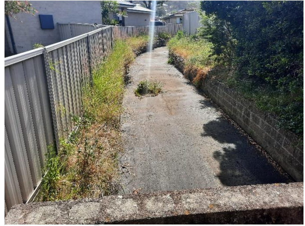
Photo 22: Concrete-lined open channel upstream of Seaman Avenue
