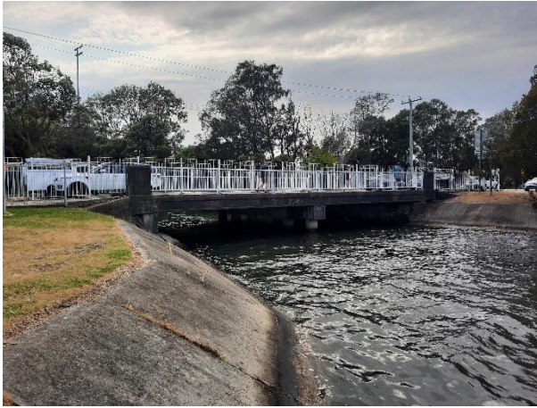
Photo 9: The Esplanade bridge over North Creek
