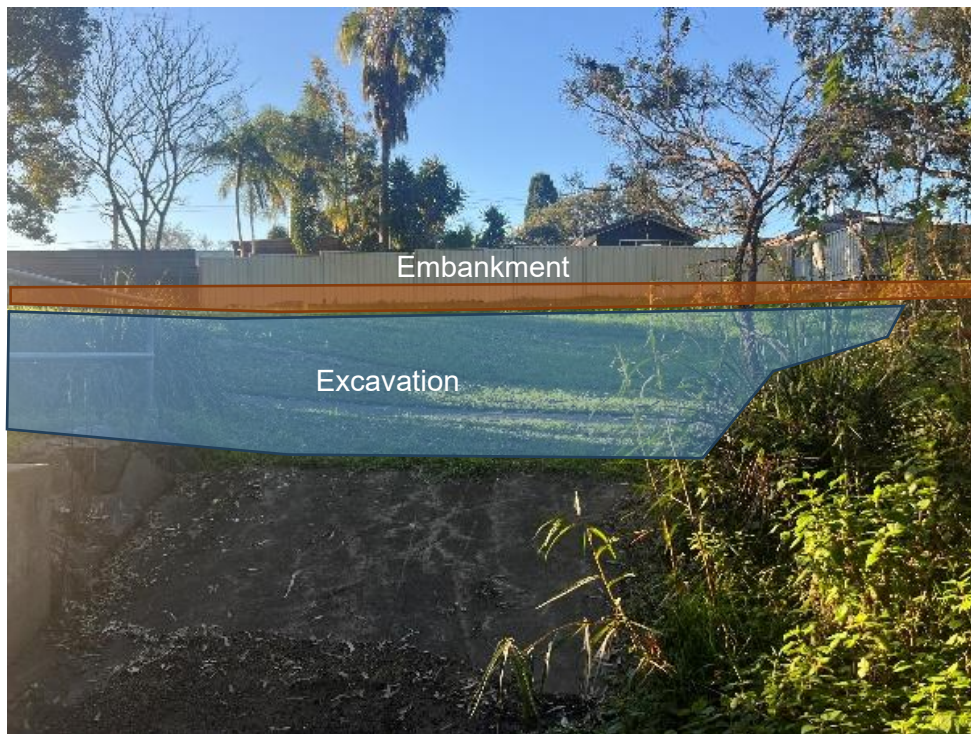
Photo 41: Wilton Close Reserve Proposed Embankment and Excavation, looking north from the culvert inlet
