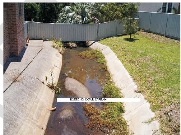
Photo 14: Example of a fence crossing the King Street Branch ( Reference 5 )
