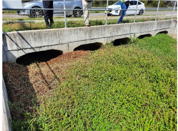
Photo 18: Biddabah Creek crossing Windross Drive
