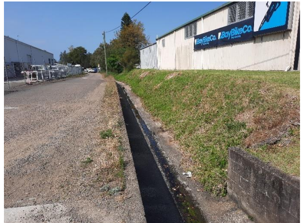
Photo 16: Concrete lined open channel downstream of Lakelands Pond
