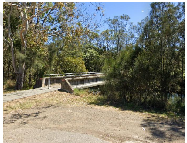
Photo 8: North Creek at John Street ( Google Street View )
