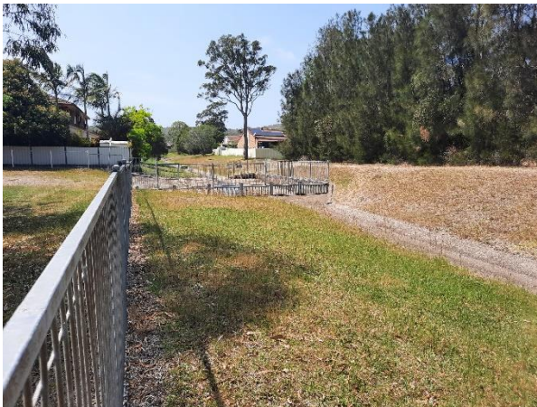
Photo 26: Looking upstream over New York Avenue GPT on Vermont Place Branch
