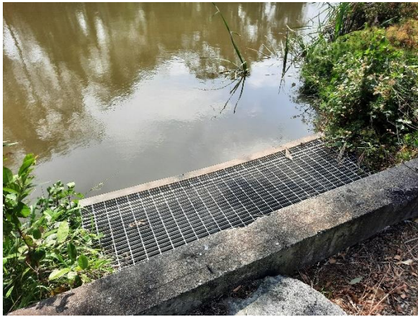
Photo 15: Lakelands Pond surcharge pit
