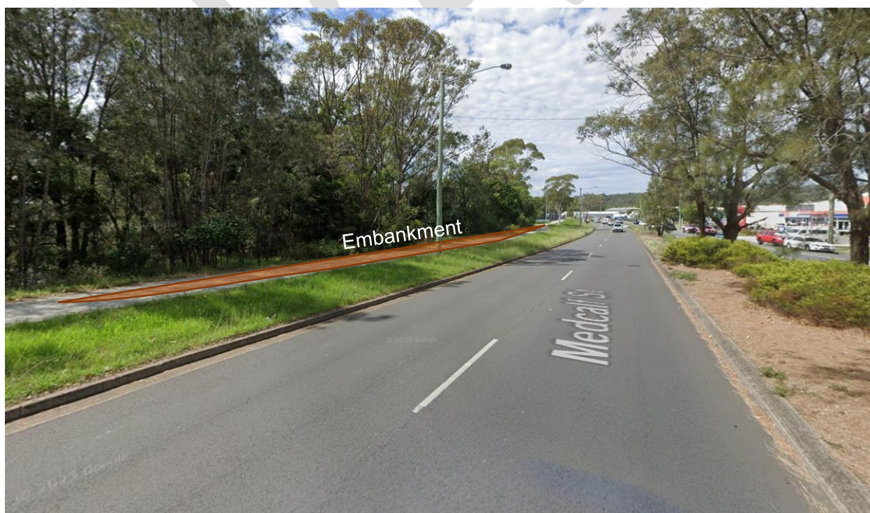
Photo 38: Lakelands Pond Proposed Embankment (Source: Google Street View)
