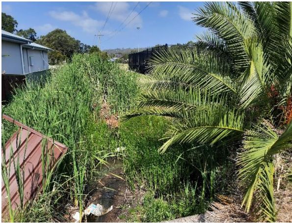
Photo 23: Open channel downstream of Seaman Avenue
