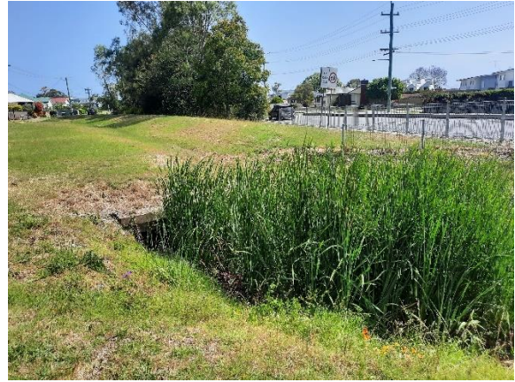
Photo 12: Drainage swale upstream of King Street
