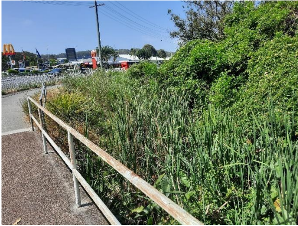
Photo 3: North Creek upstream of King Street
