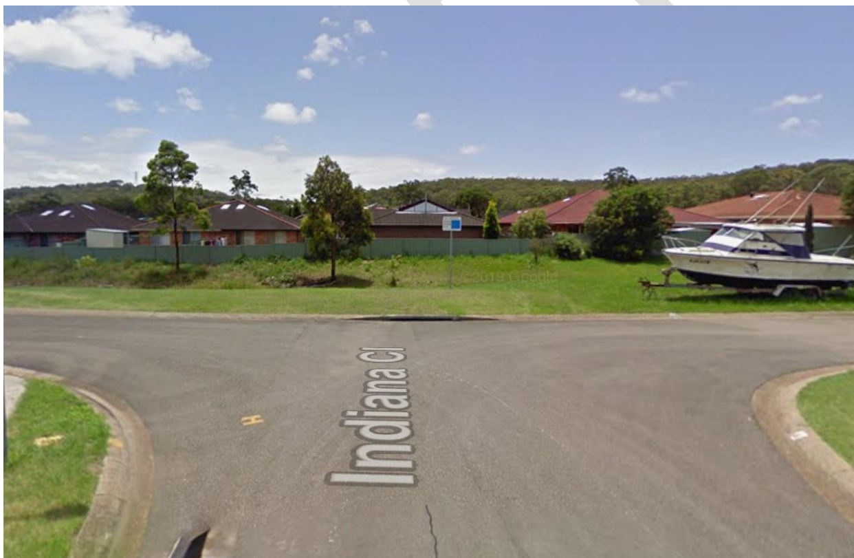
Photo 37: Indiana Close low point at the end of the road, with an embankment restricting overland flows to the flow path ( Source: Google Street View )
