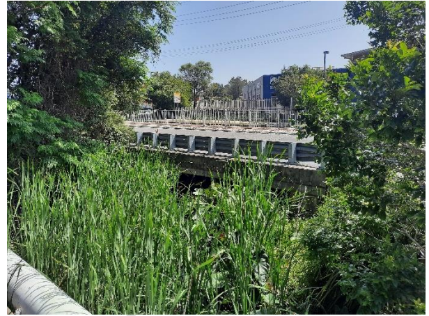
Photo 4: North Creek crossing King Street
