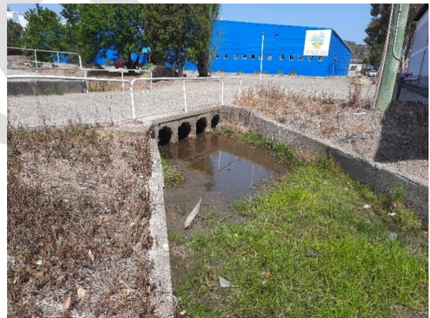
Photo 2: Section of concrete channel through the Hillsborough Road commercial area
